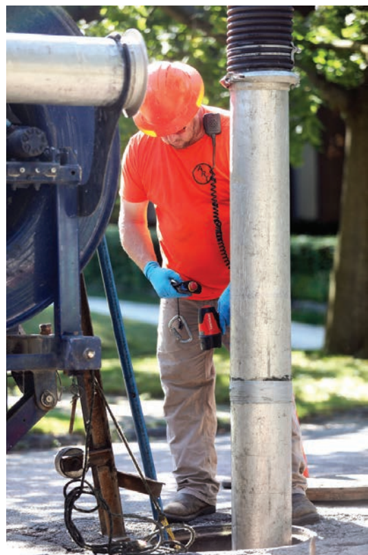
Justin Parnham keeps on eye on a manhole while remotely operating a sewer cleaner.
